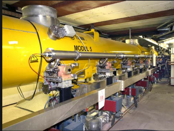
a) Superconducting modules
