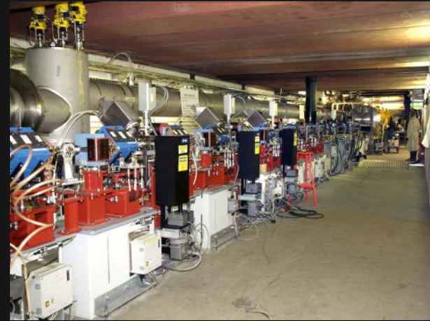
b) Beam line with diagnostic system
