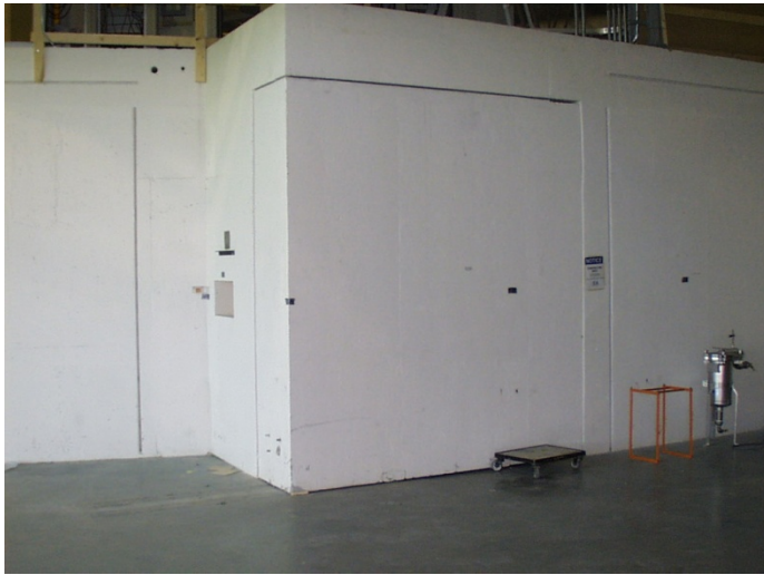
Storage Ring Outer Wall
