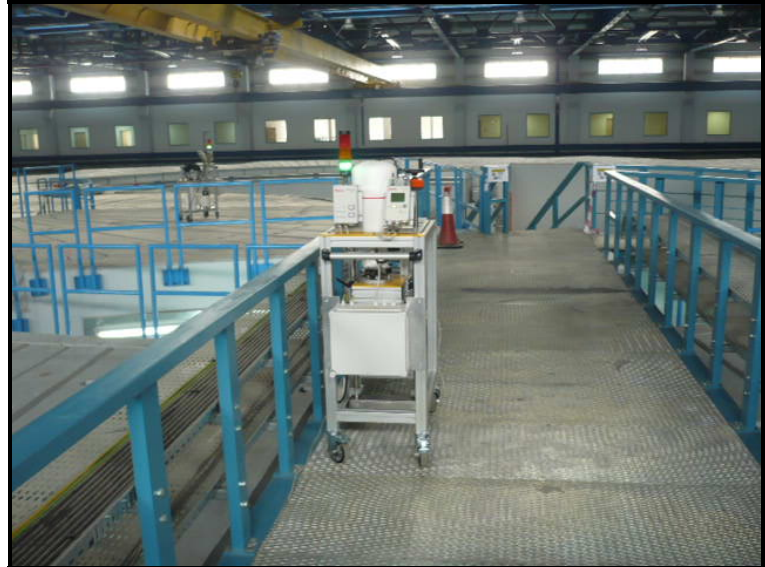
Fig: 2c. On both bridge and Microtron roof.
