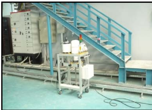
Fig: 2d. In the main service area.
